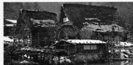
Farm houses in the gassho-zukuri (praying hands) style at Hida Folklore Village in Takayama. The steep roofs of the three-story structures were designed especially for mountain areas to keep snow from piling up.
